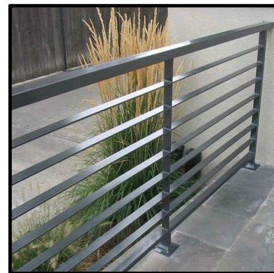
9. FLOOR MOUNTED METAL BALCONY RAILING
